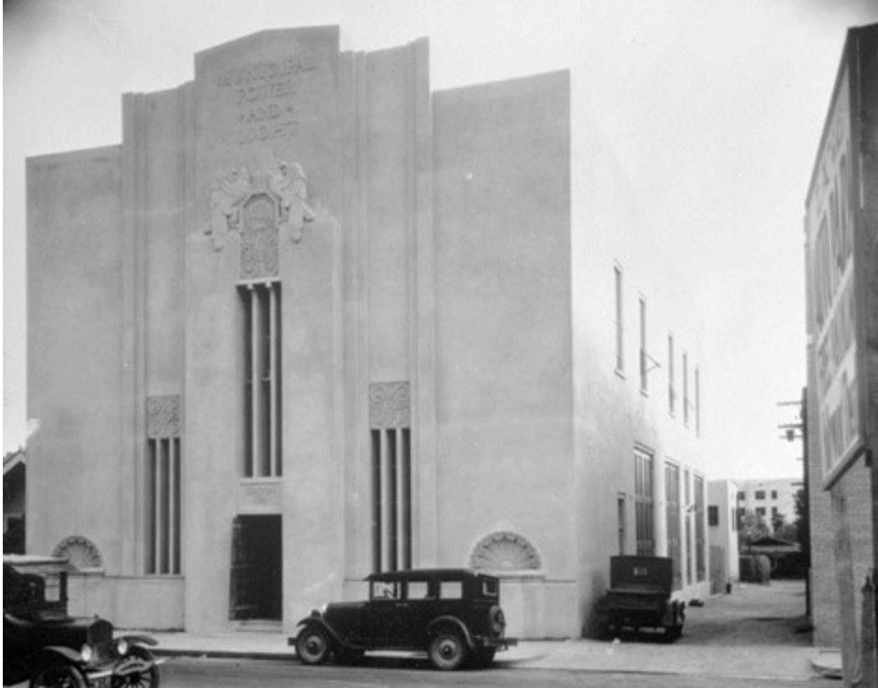
Distribution Station No. 10 in 1933, the year it was put into service. Notice the sign at the top that reads "Municipal Power and Light." (Photo courtesy of Water and Power Associates)
