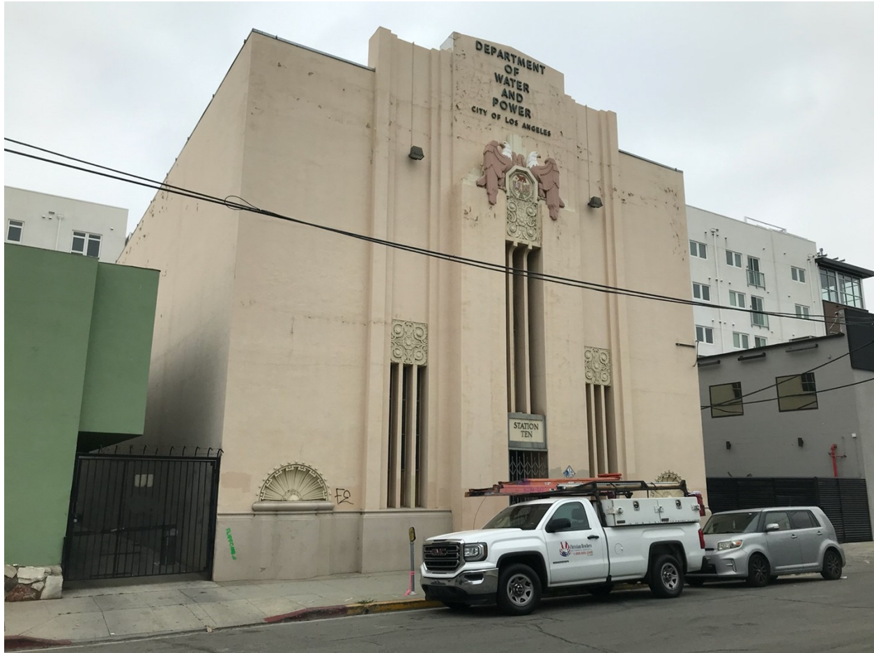
Distribution Station No. 10 is on Hawthorn Avenue between Highland Avenue and McCadden Place. (Photo by Steven Herrera.)
