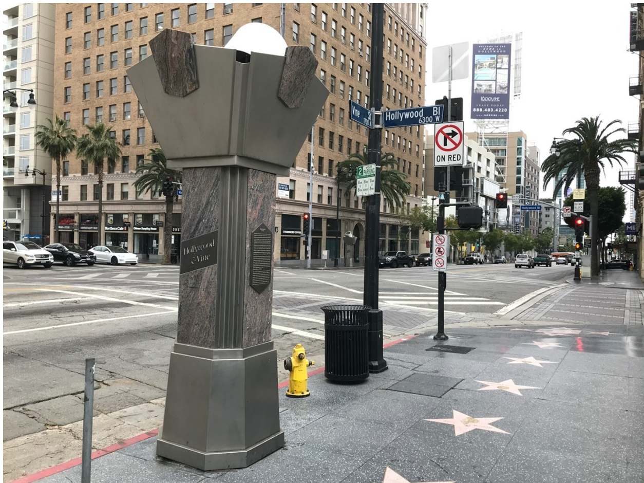
Each SkyTracker light is perched atop a ten-foot-tall column made of metal and marble. (Photo by Steven Herrera)
