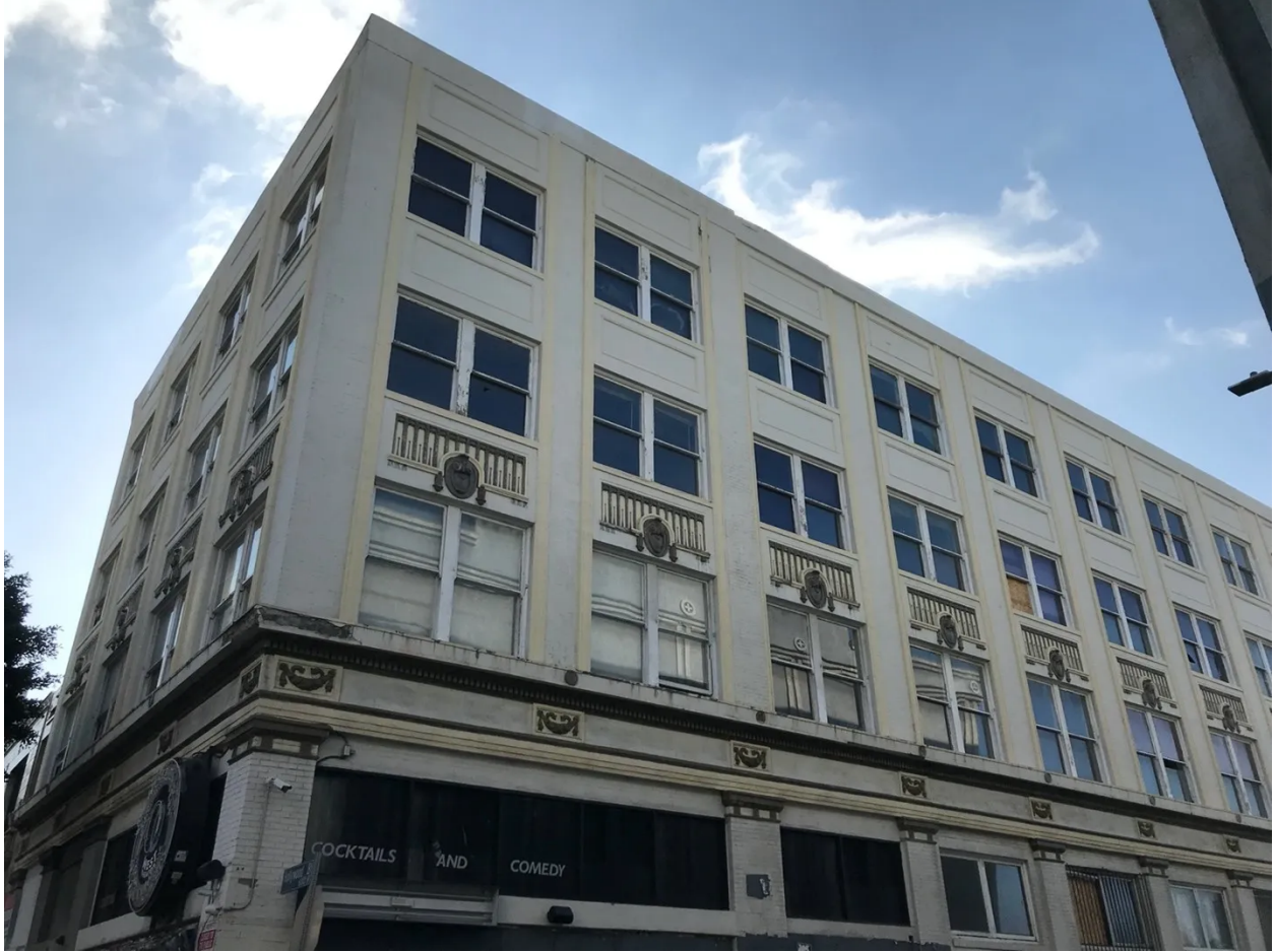
The Palmer Building façade facing Cosmo Street. (Photo by Steven Herrera)
