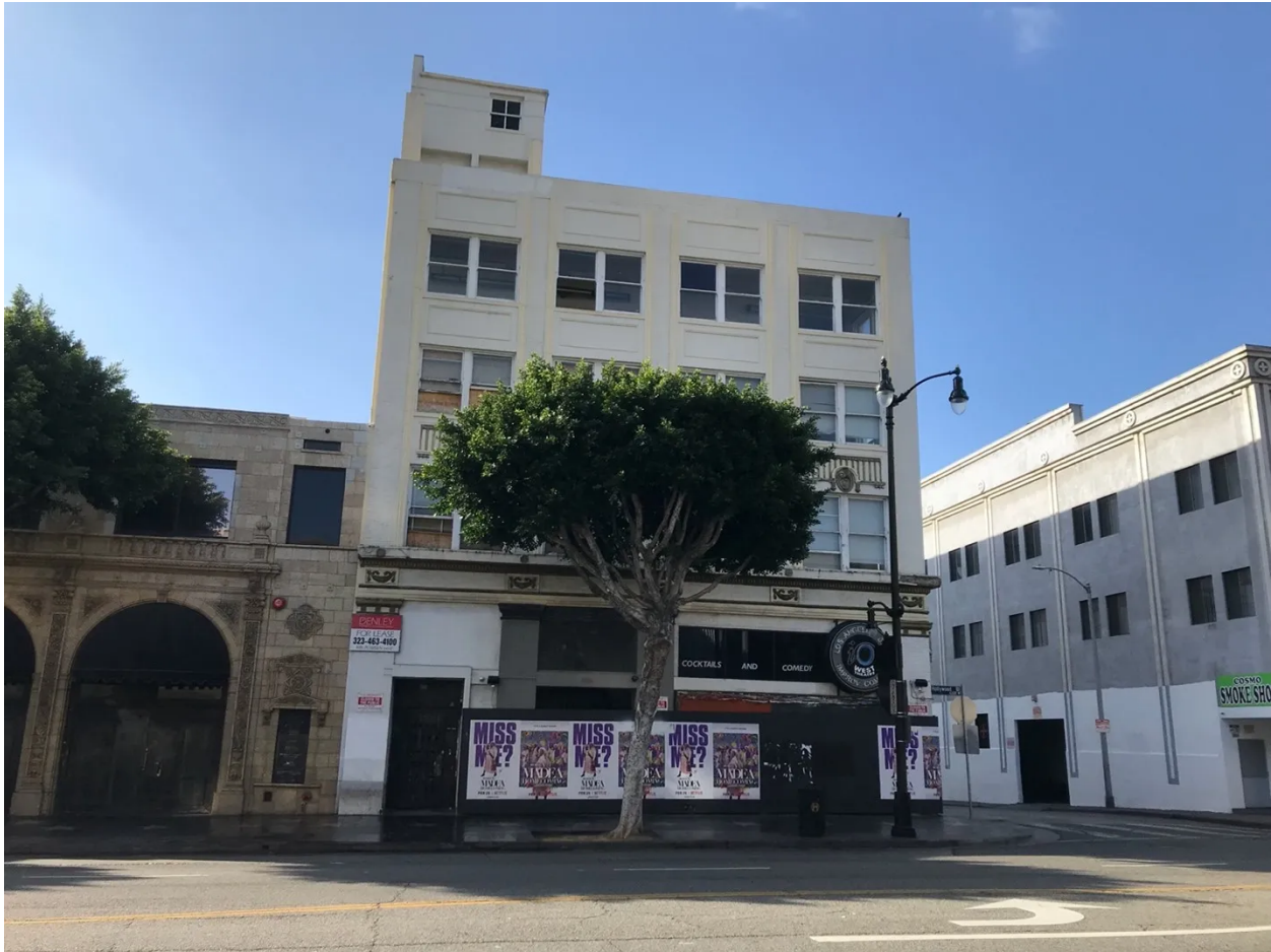
The Palmer Building is located at 6360-6366 Hollywood Boulevard. (Photo by Steven Herrera)
