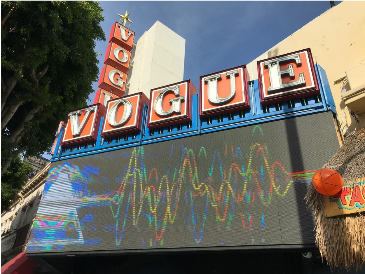
The building currently features a digital marquee for advertising. (Photo by Steven Herrera)
